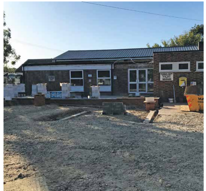
The foundations for the new extension to the village hall
