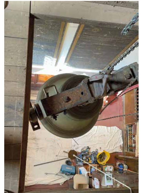
The bell going through the second trap door
