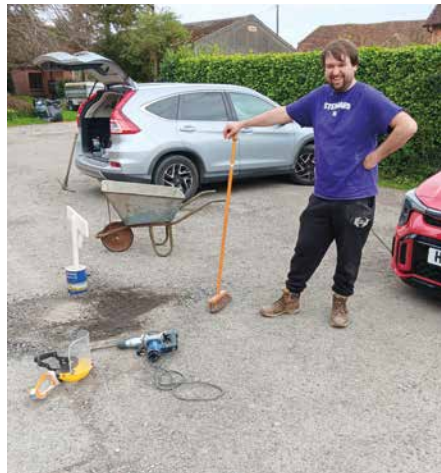
One hole nearly done
